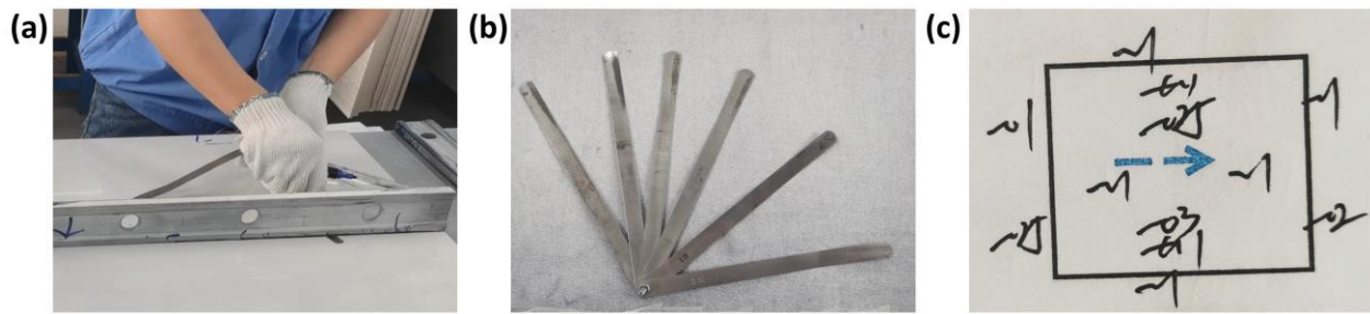
Fig. 2. (a) Illustration of manual inspection; (b) Feeler gauge used to measure the gap width; (c) Recordings of manual inspection results.
